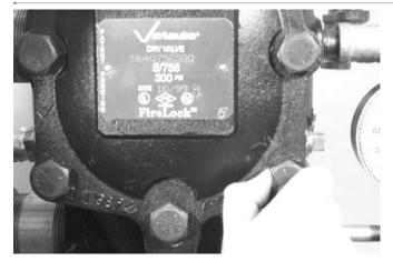
4. Align the cover plate/cover plate gasket to the valve. Make sure the clapper spring's arms are rotated to their installed position. Tighten all cover plate bolts into the cover plate/valve body.
