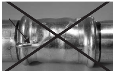
5 - Press Resulting from Improperly Maintained Press Jaws
