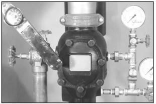
**5.** Torque all cover bolts in an even, crossing pattern. Refer to the "Cover Bolt Torque Requirements" chart on this page for the required torque values. DO NOT over-tighten the cover bolts.
