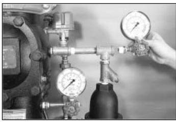
**5.** Install the reducing bushing/nipple/gauge valve assembly into the tee coming from the Series 75D Water Column Kit.
