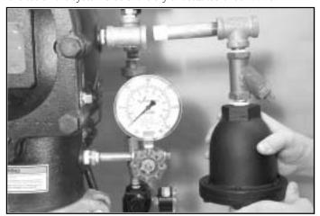
**4.** Install the Series 75D Water Column Kit into the tee where the gauge valve assembly was removed in step 3.
