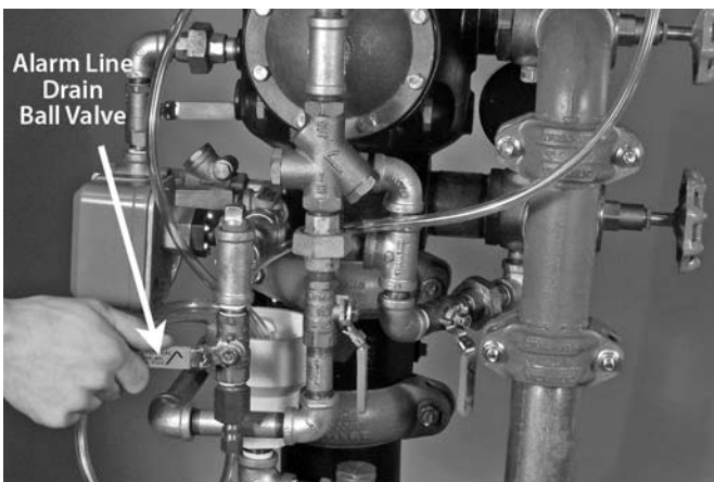
9. Close the alarm line drain ball valve.
