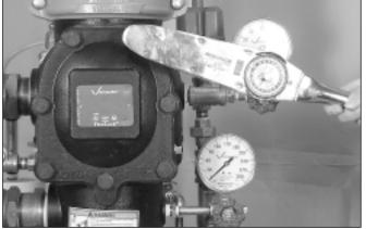
**3.** Tighten all bolts using an even pattern. Tighten the bolts to the proper torque per the chart below. Do not over-tighten.
