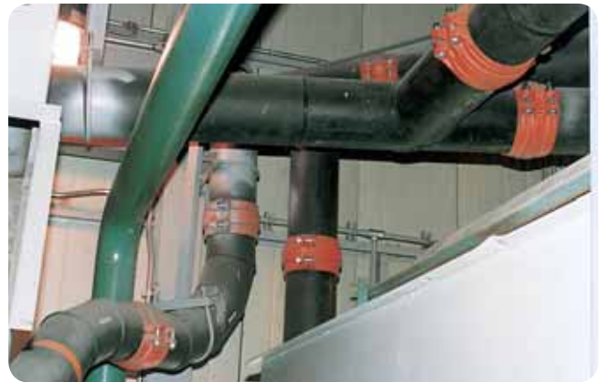
Use of HDPE for in-plant services allows pipe rotation and re-use for additional cost savings.
