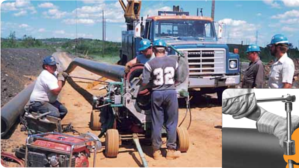
Expensive equipment and higher labor costs are involved when joining HDPE pipe using traditional butt welding methods.
