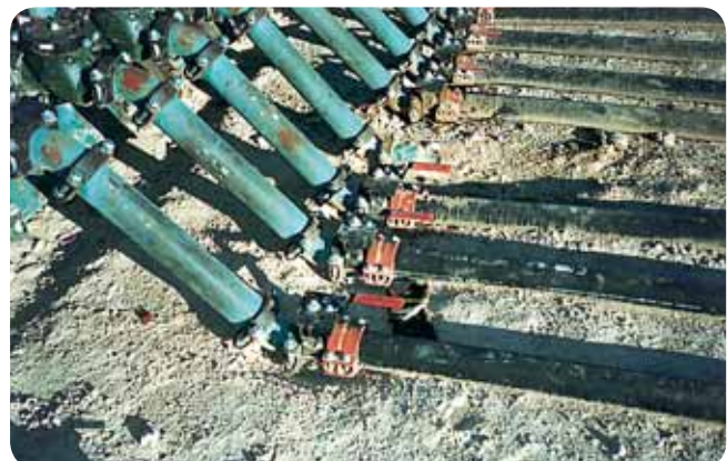
HDPE transition coupling provides a direct connection from HDPE to grooved IPS pipe, valves and fittings.
