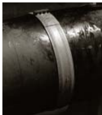
74" ExE T1 RC on steel pipe.
