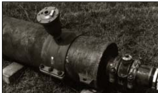
16" FxF T1 Outlet Coupling on spiral weld steel pipe.
