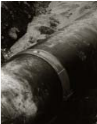
54" ExE T2 RC on HDPE pipe.
