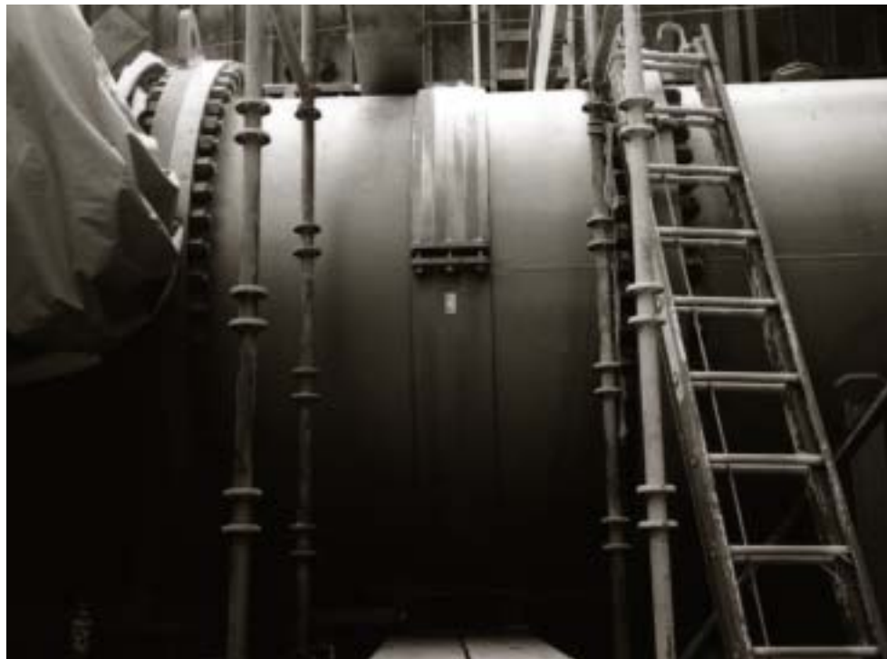
86" ExE T2 on steel pipe.
