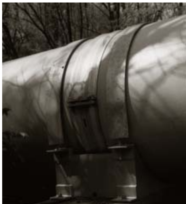
54" ExE T1 on FRP pipe.
