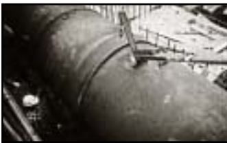
72" ExE T1 on steel pipe.
