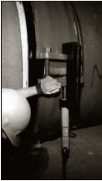
Hydraulic Closure Tool on FxF T2 on cement coated steel pipe.
