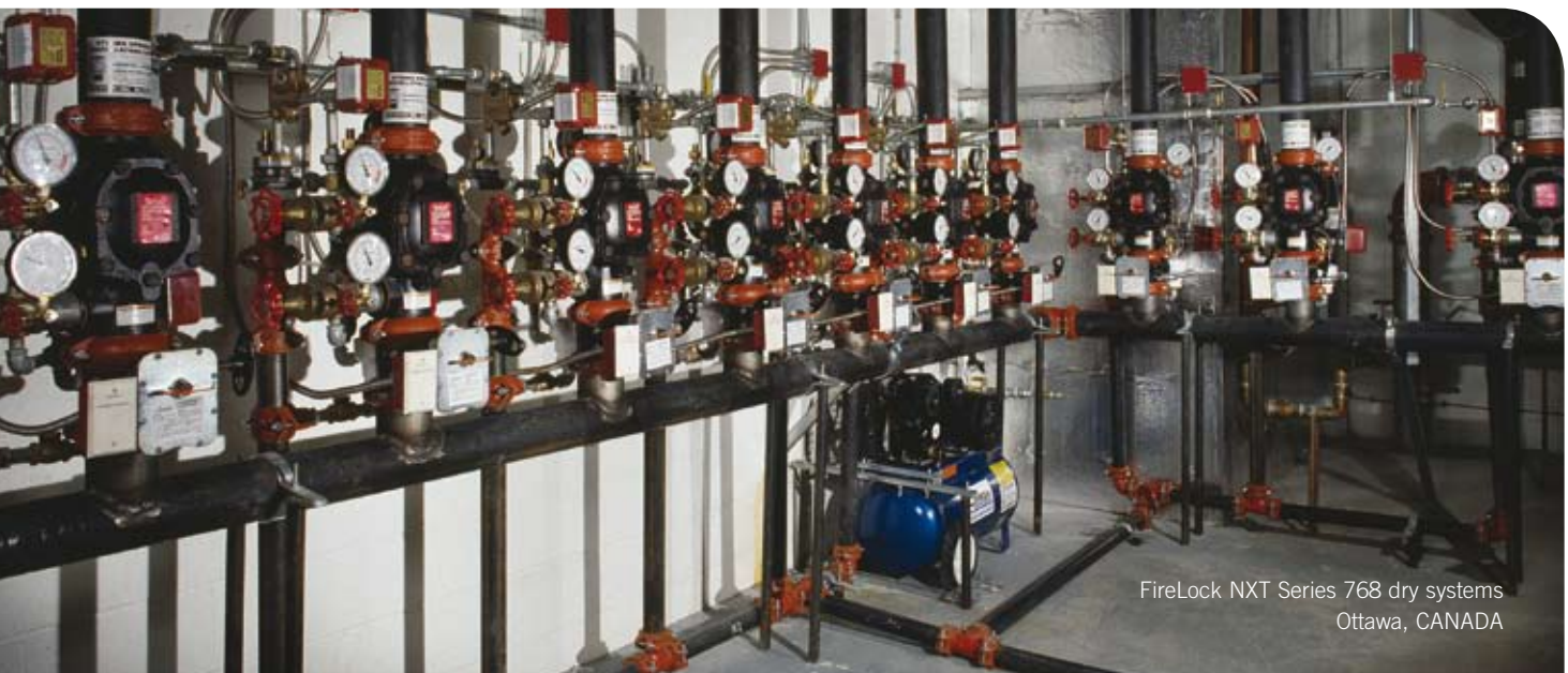
FireLock NXT Series 768 dry valve shown
